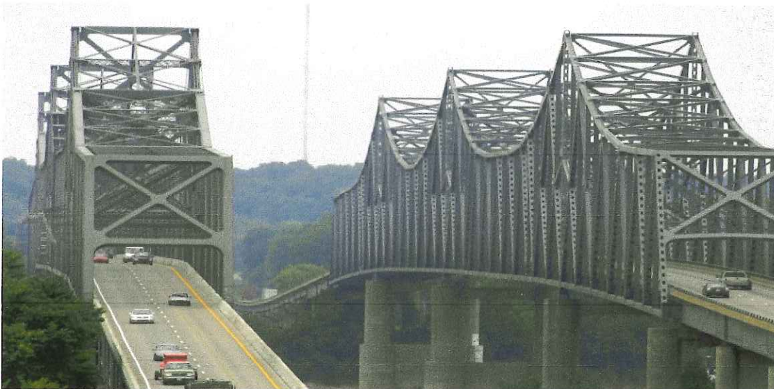
US 41 Twin Bridges
