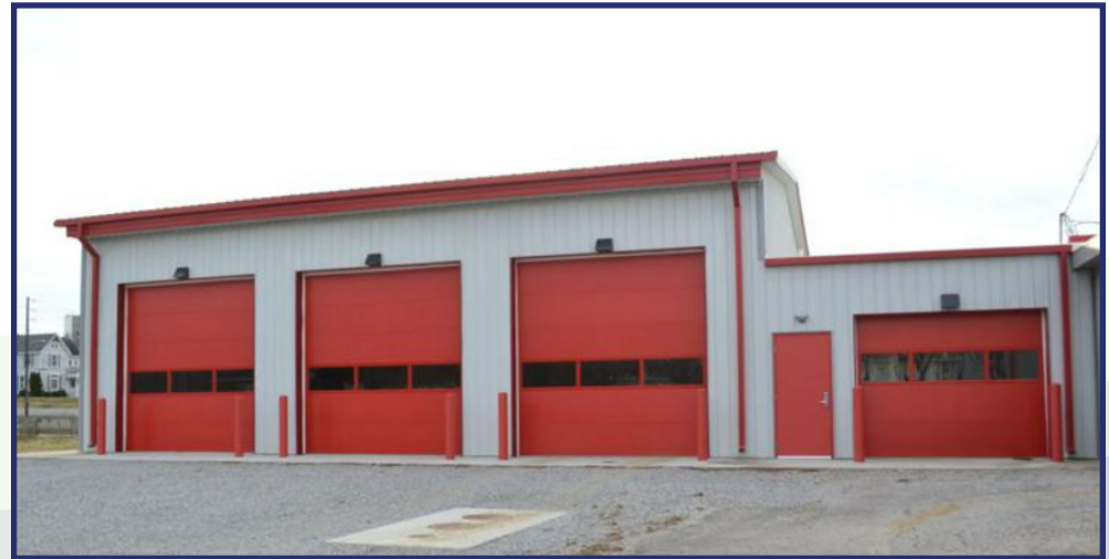
New Livermore fire station SOURCE: Freddie Bourne/McLean County News
