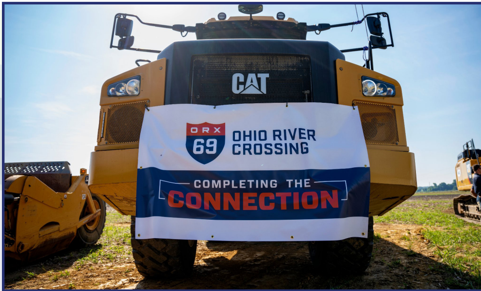
Groundbreaking of the I-69 Crossing Project
