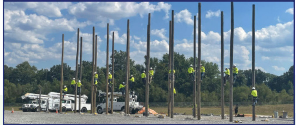
Utility lineman training at the Lisman Workforce Complex
