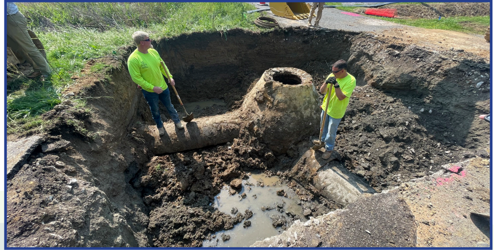
Unearthed manhole in Morganfield as part of the Job Corps Sanitary Sewer Rehabilitation. SOURCE: GRADD
