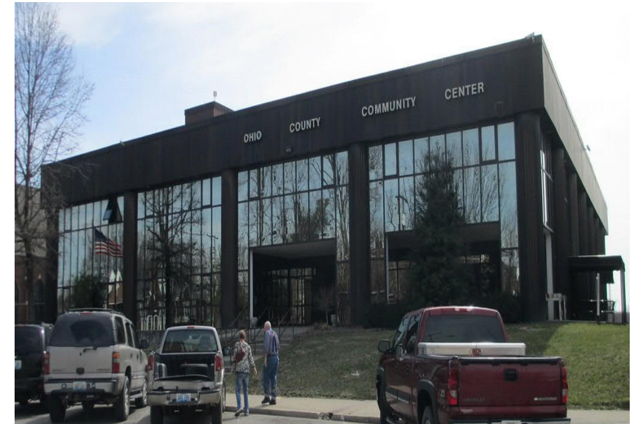
Figure 1: The Ohio County Community Center
